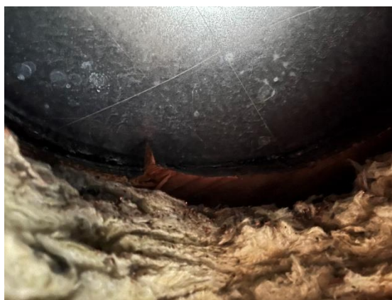
Billede 12, viser tagreparation.
